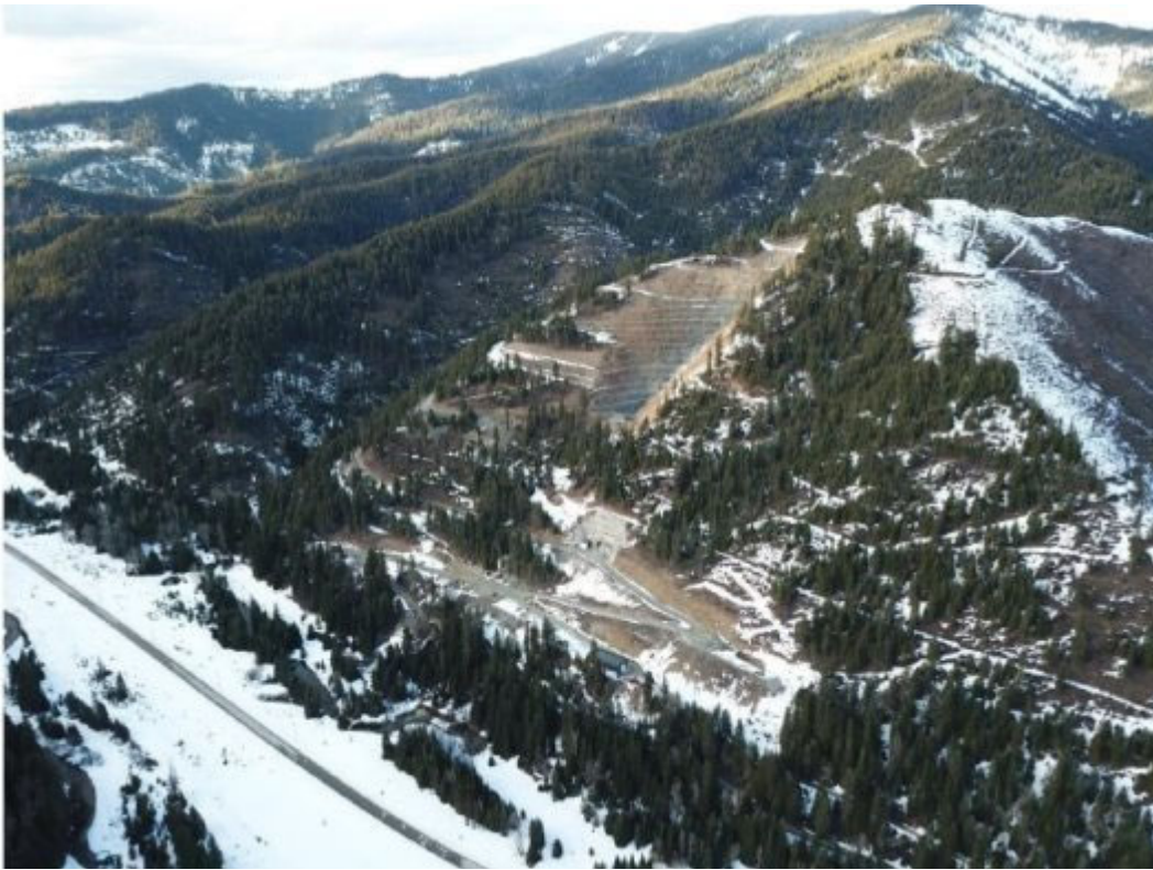
Figure 2 – Aerial Photo of Golden Chest Mine in February 2020
