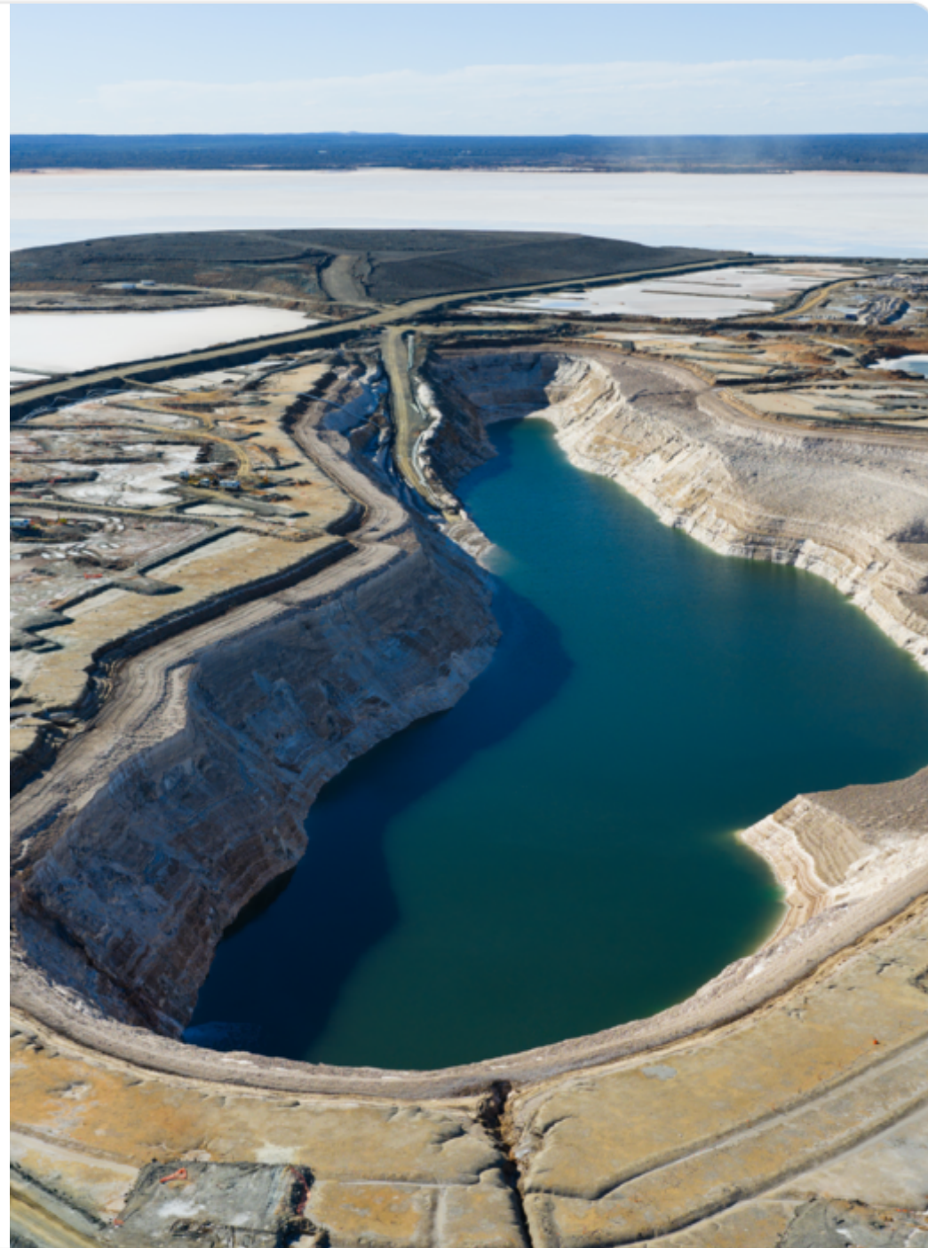
St Ives tailings facility
